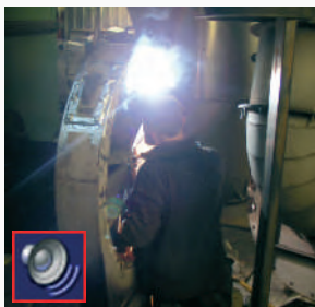
Jim welds 22dB attenuator inside the burner fan ...
